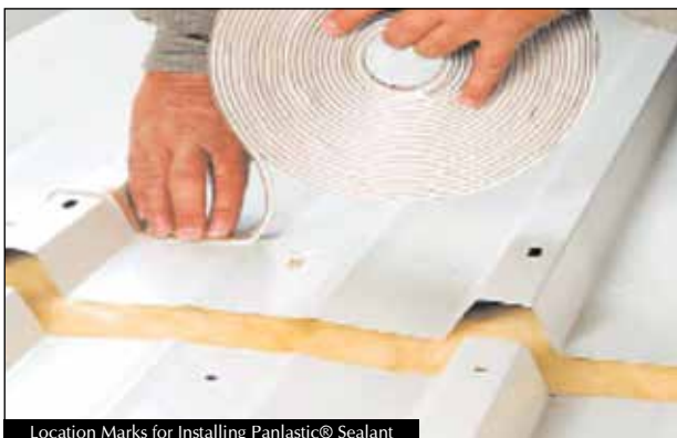
Location Marks for Installing Panlastic® Sealant
